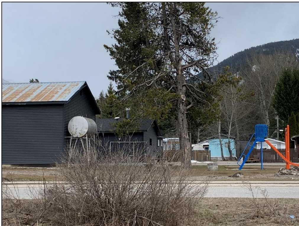
Photo 22: An AST observed east of the Site across Cokato Road.
