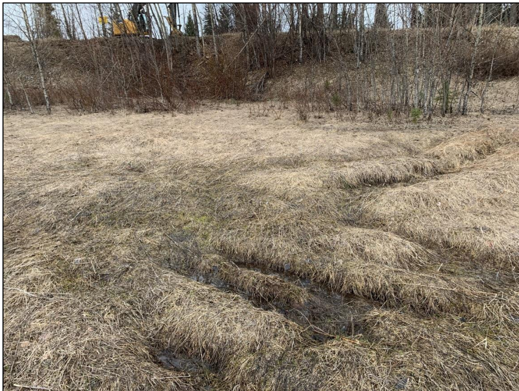
Photo 14: Rill erosion observed near the center of the Site.
