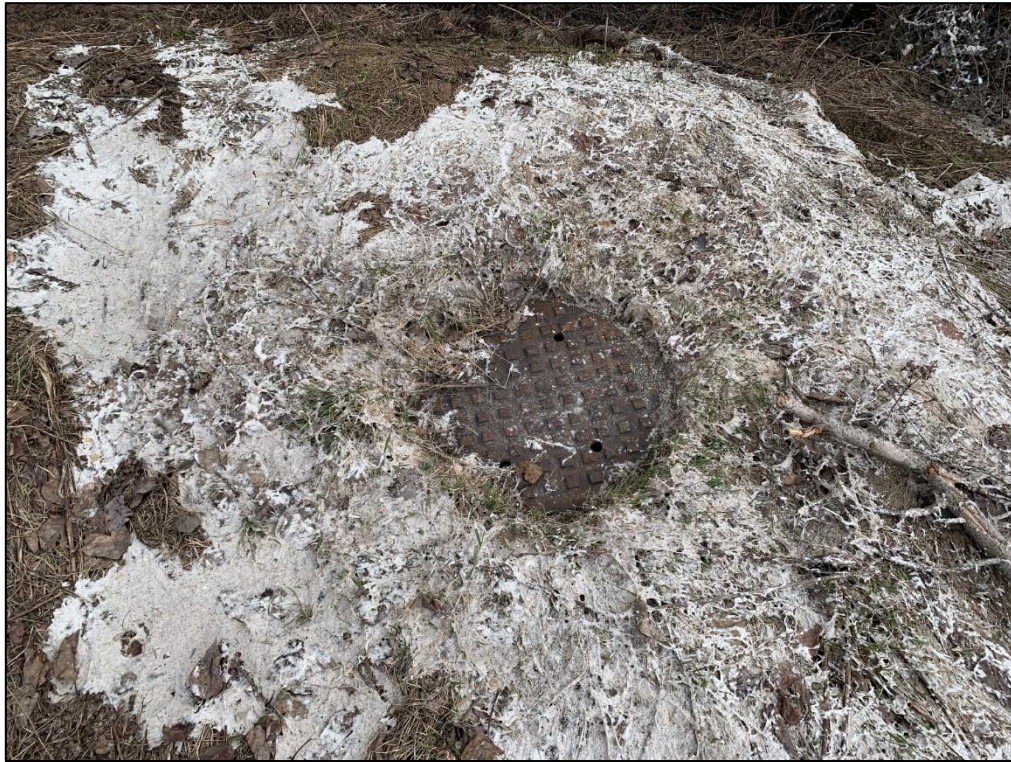
Photo 9: A drain observed on-Site with dry foam material surrounding it.
